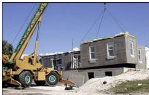
photo by Glenn Tucker Modular Housing A crane places pieces of a modular house that was raised in a single day in Hamilton.
